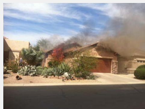
Feb. 21 - Stone Circle Ln. in Peralta Firefighters encountered barricaded furniture and other intentional hazards while fighting this fire. The resident was later apprehended by PCSO after reportedly setting this fire, discharging weapons, and fleeing the scene.
