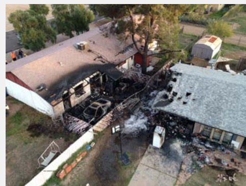
Feb. 27 - 1700 block of W. 9 th Ave. The cause of the fire was determined to be a 7-year-old playing with a lighter. Due to heavy fire load and wind, the fire spread to the adjacent duplex.
